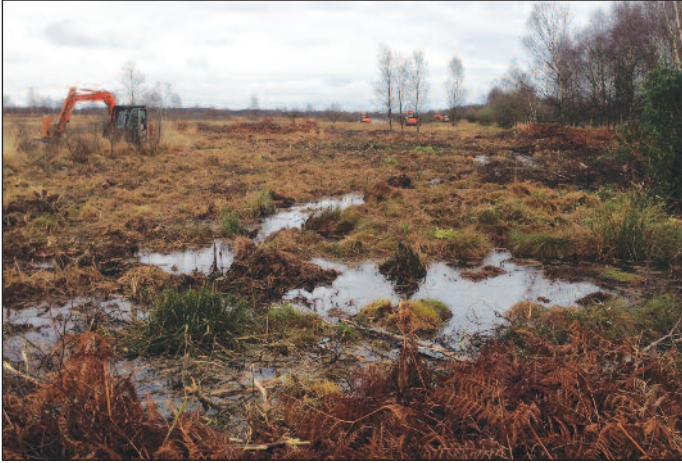
Above: Excavators mulching taller patches of birch around the site margins.
